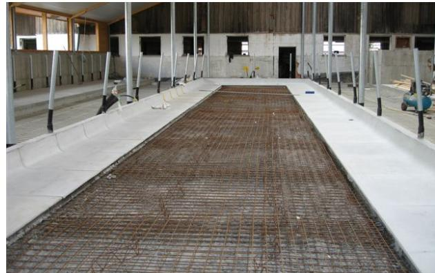
3. Secure the trough base with mortar.
